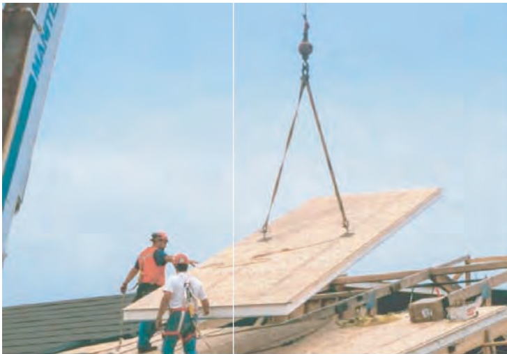
Lifting a SIP with Lifting Plates
