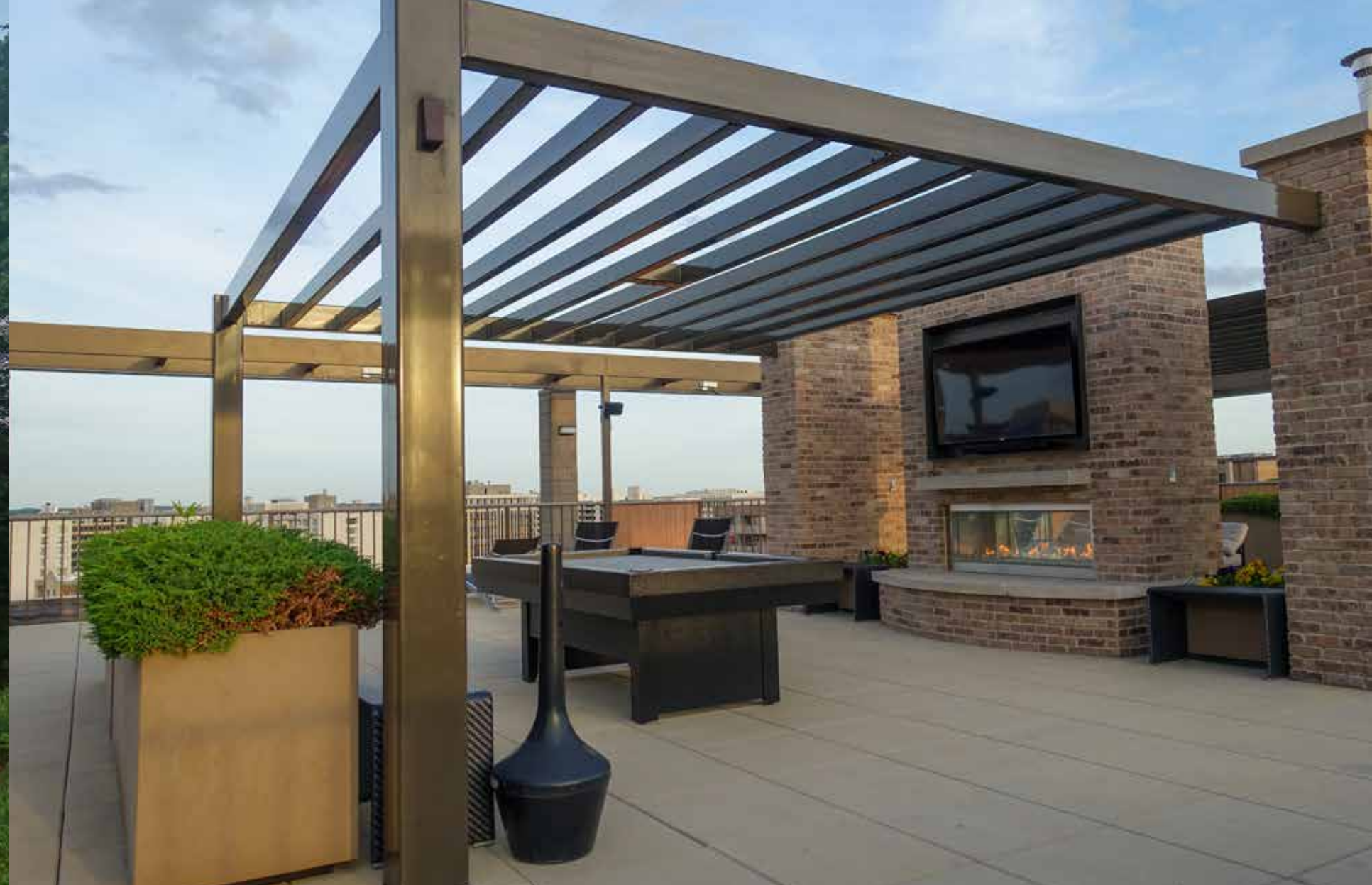
Rooftop Patio - Union City, NJ 20'x37' Rooftop Trellis 37
