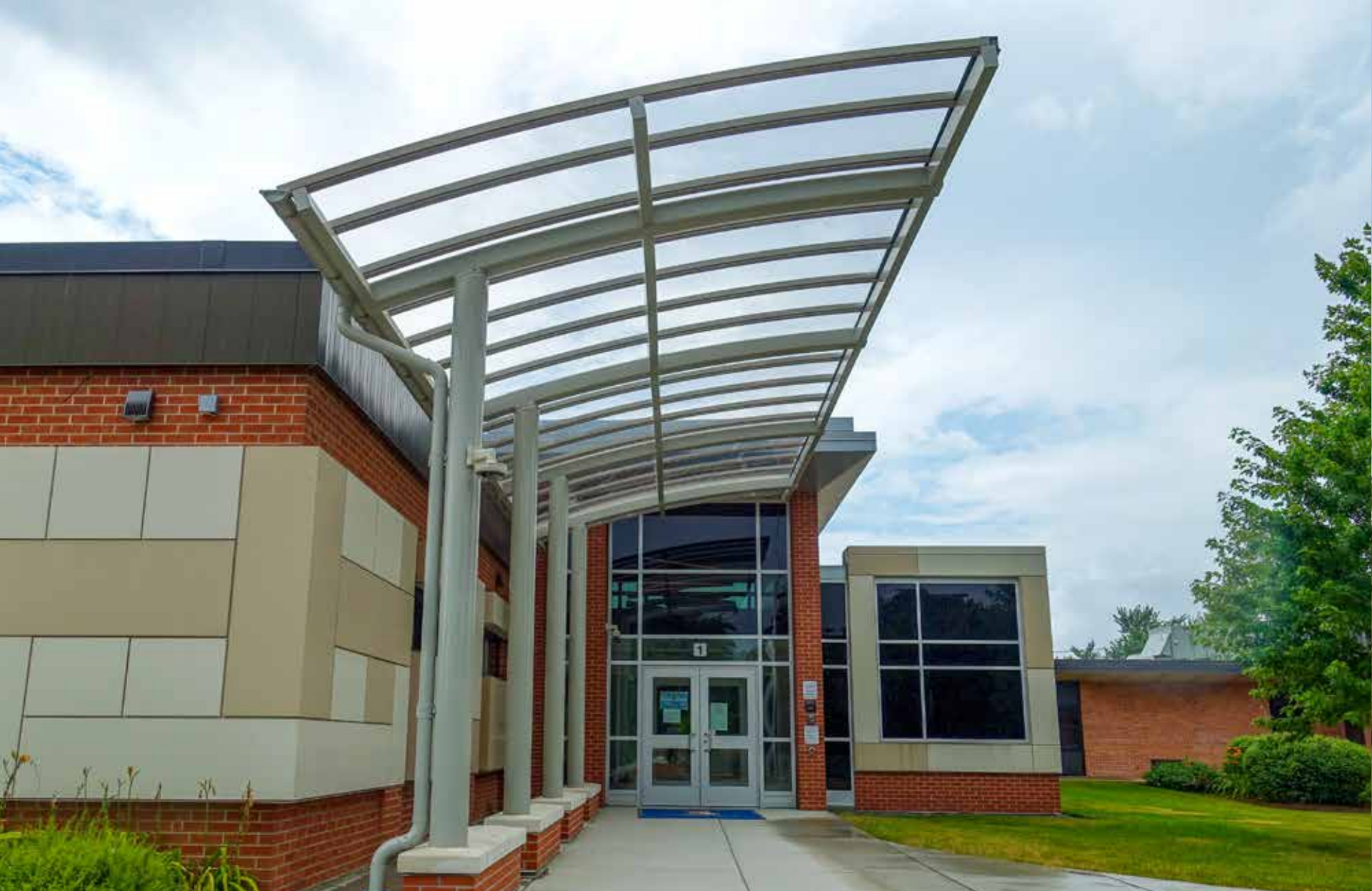
Elementary School - Carol Stream, IL 13'x35' Entrance Canopy
