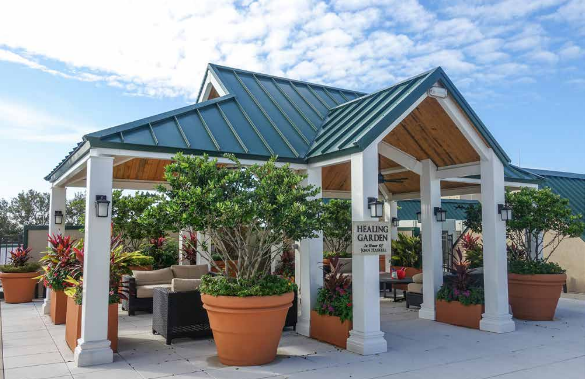
Ronald McDonald House - Jacksonville, FL 28 17'x29' Rooftop Pavilion
