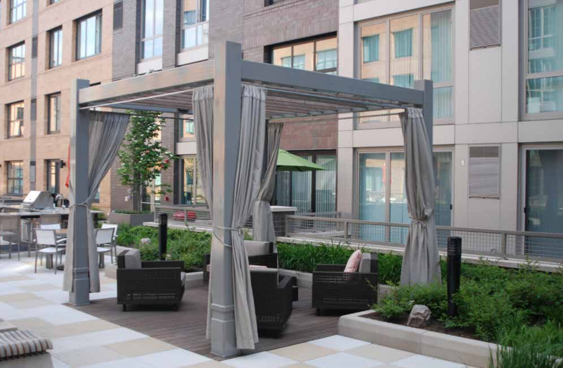
Residential Building - Weehawken, NJ 34 12'x12' Rooftop Trellis
