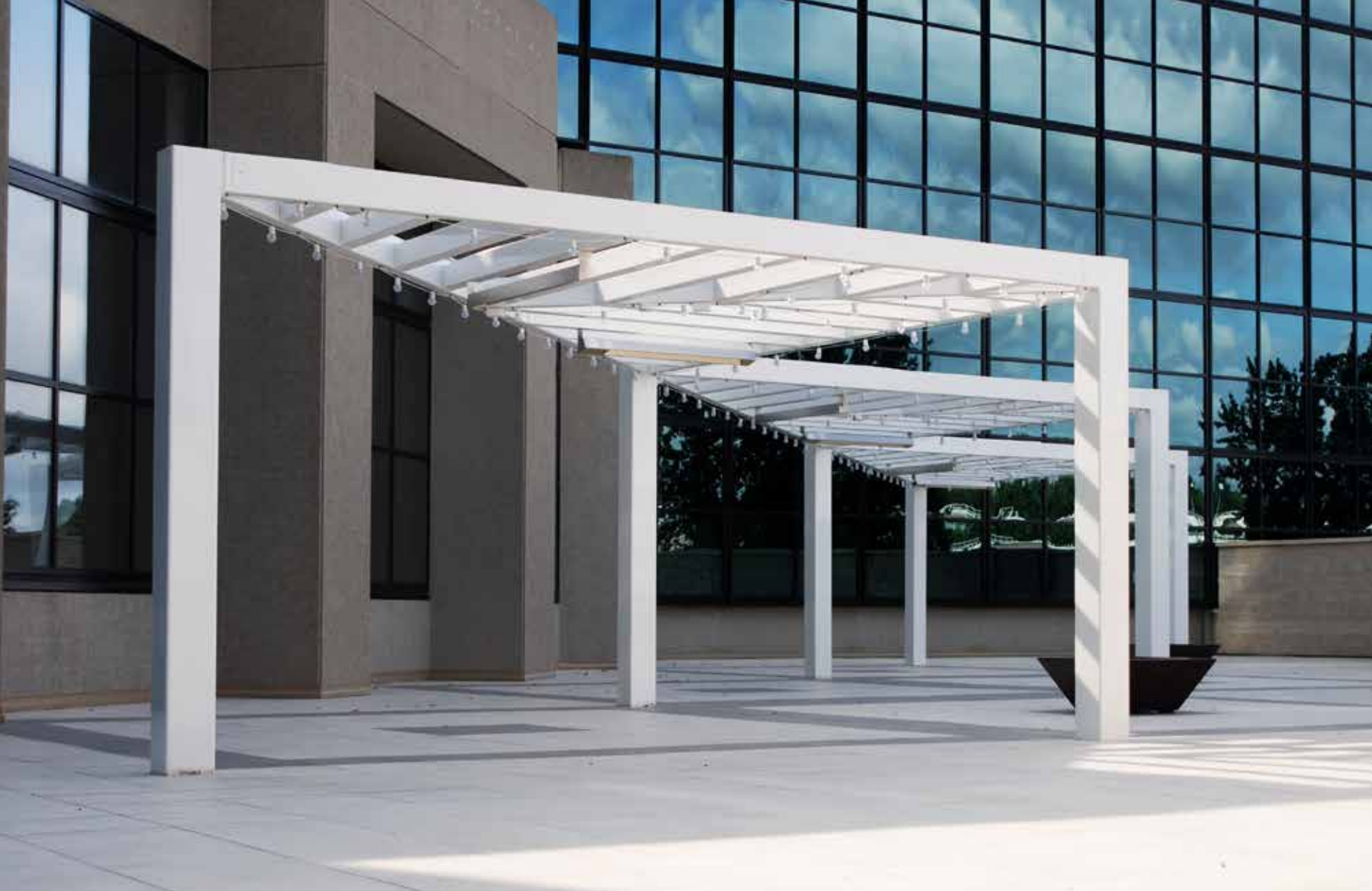
Corporate Rooftop - Falls Church, VA 15'x85 Trellis 33
