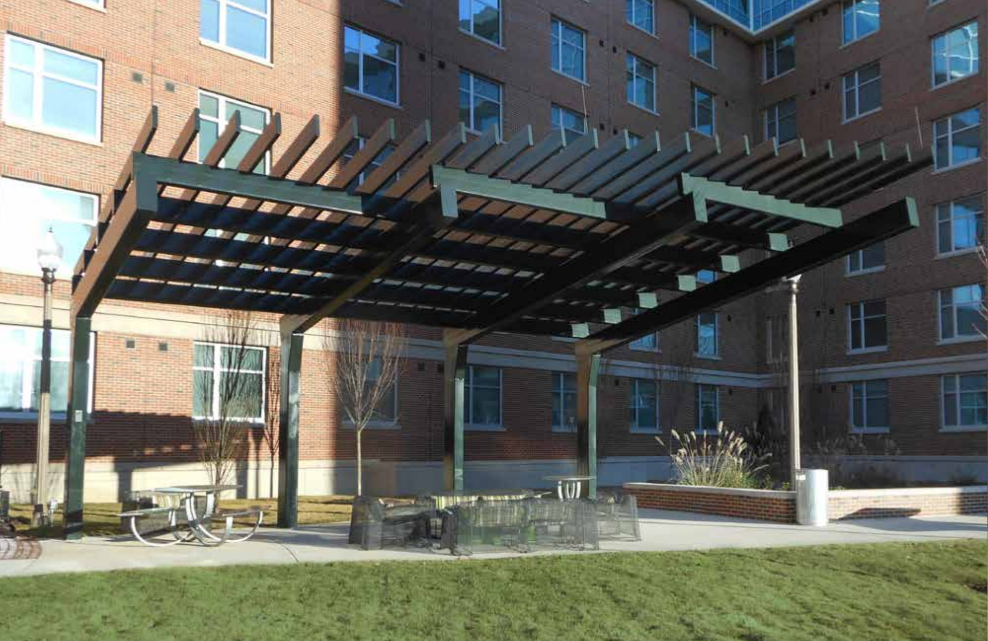
Univ. of Alabama Residence Hall - Birmingham, AL 32 30'x25' Trellis
