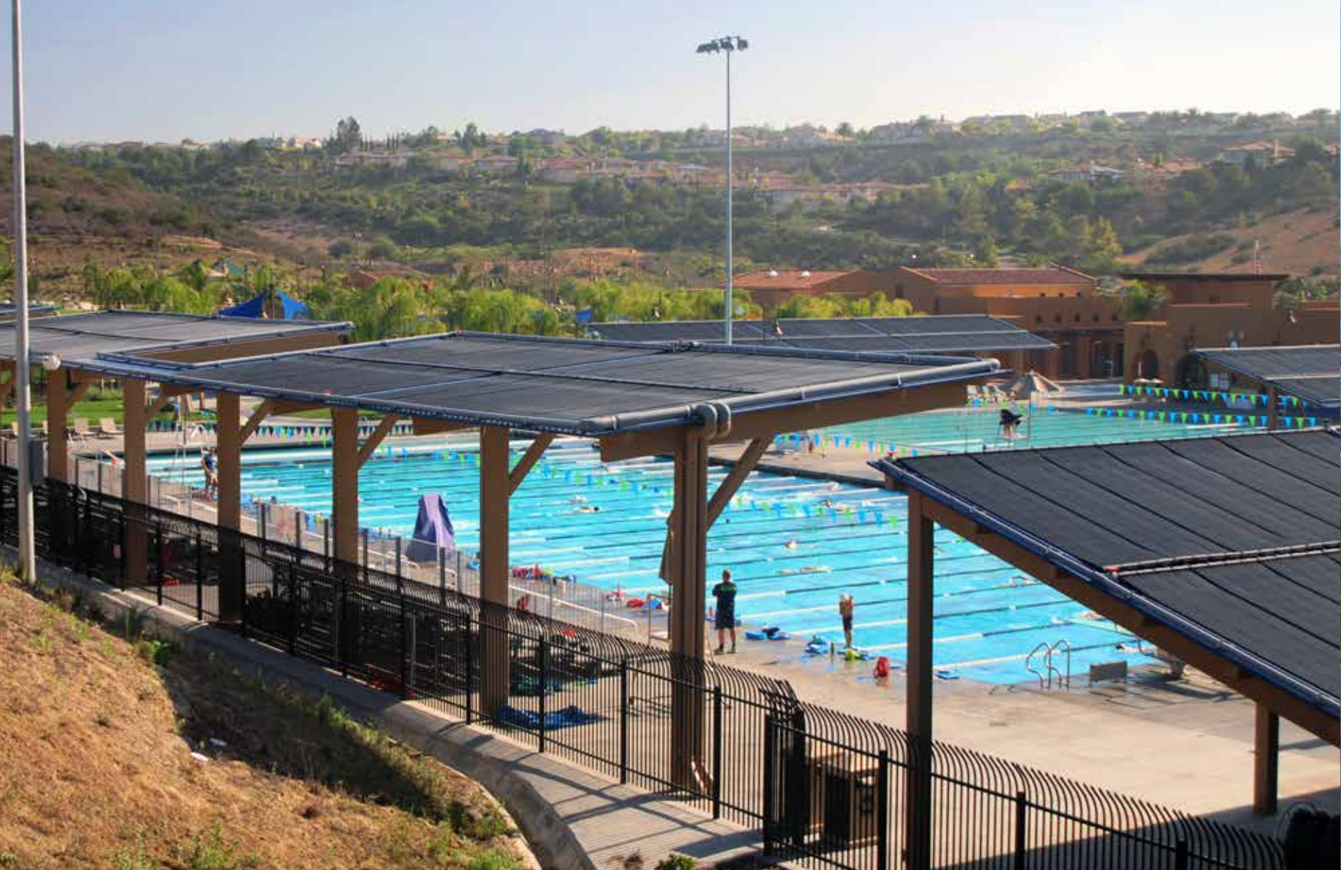
Alga Norte Park - Carlsbad, CA 18 Monoslopes w/ solar panels (by others)
