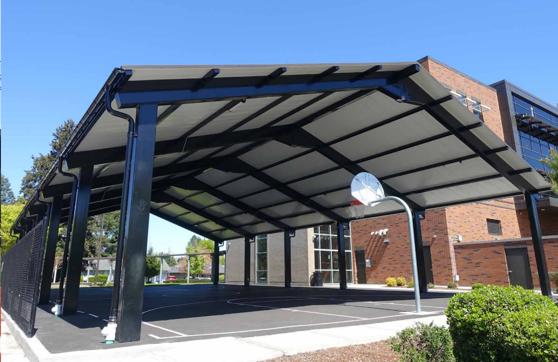
Hela Evergreen School - Vancouver, WA 19 50'x84' Pavilion
