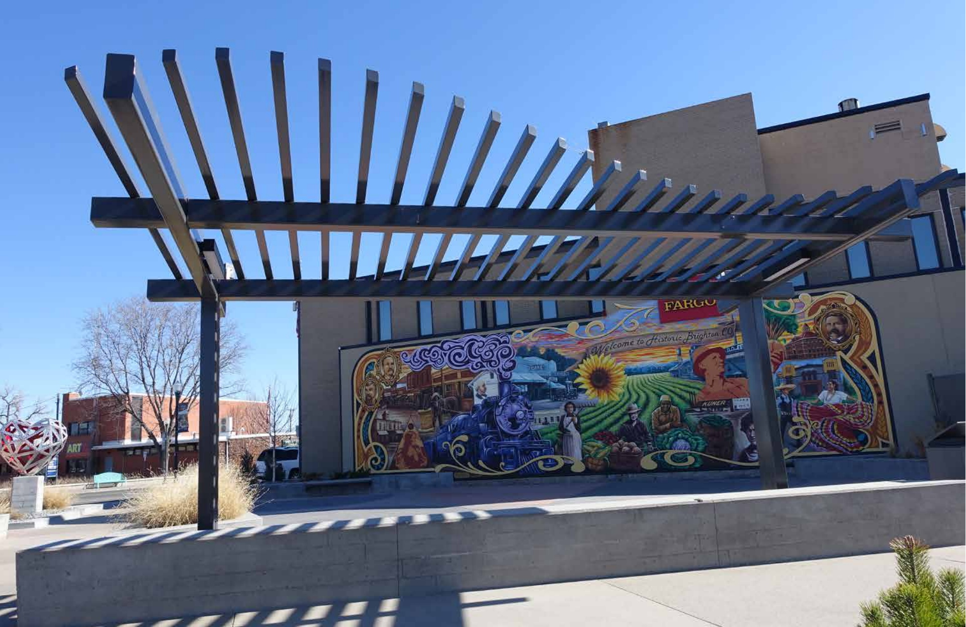
Shopping Center - Denver, CO 28 14'x25' Trellis
