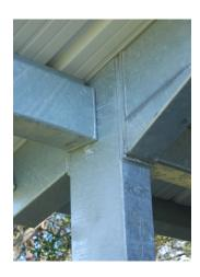
Galvanized - A basic, long-accepted method of protecting steel from corrosion, galvanizing is the process of coating steel with zinc using a hot bath process. Galvanizing is considered the best corrosion protection process available for steel components and is commonly used where exposure to salt air is anticipated. The galvanizing process results in a random, spangled finish that can also have alternating areas of haze and sheen.
