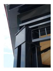
Poli-5000<sup>®</sup> Powder Coat - The most durable powder coat finish system in the industry. Steel is shot blasted to a near white condition, given a phosphate wash, coated with an epoxy primer, and then followed with a coat of polyester TGIC powder formulated for maximum UV protection, adhesion, and fade resistance. The Poligon Poli-5000 process is a completely in-house system and is available in a wide range of smooth, textured, and metallic colors.
