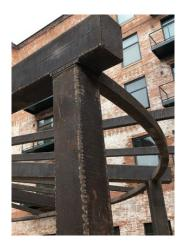
Antiquity - A Poligon finish that creates the look of time-weathered steel. Antiquity is a finish system that combines hot dip galvanizing, the best means of corrosion protection, with a secondary stain etching process that results in a varied rustic brown color. A shelter protected with the Antiquity finish will not appear new but rather as one that has been in place for decades.
