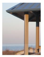
Powder Coat over Galvanized - The combination of hot dip galvanizing with TGIC powder coating combines the ultimate corrosion protection with the color selection of super-durable powder coating. This long-sought combination has been difficult to successfully achieve but a new proprietary process is now making this finish combination available. Due to the galvanizing process, there will be noticable texture areas in the final powder coat finish.
